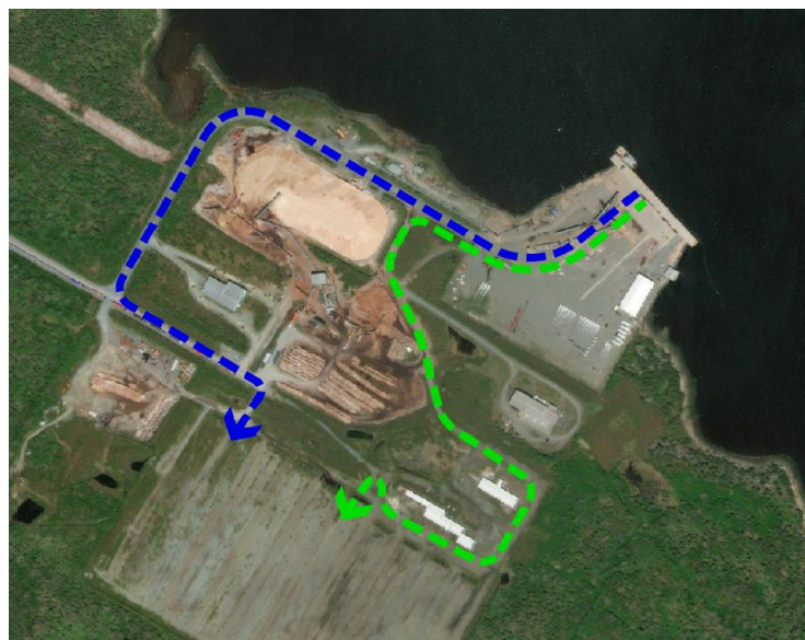
Figure 6 - Existing Route(s) to Upper Laydown Area
