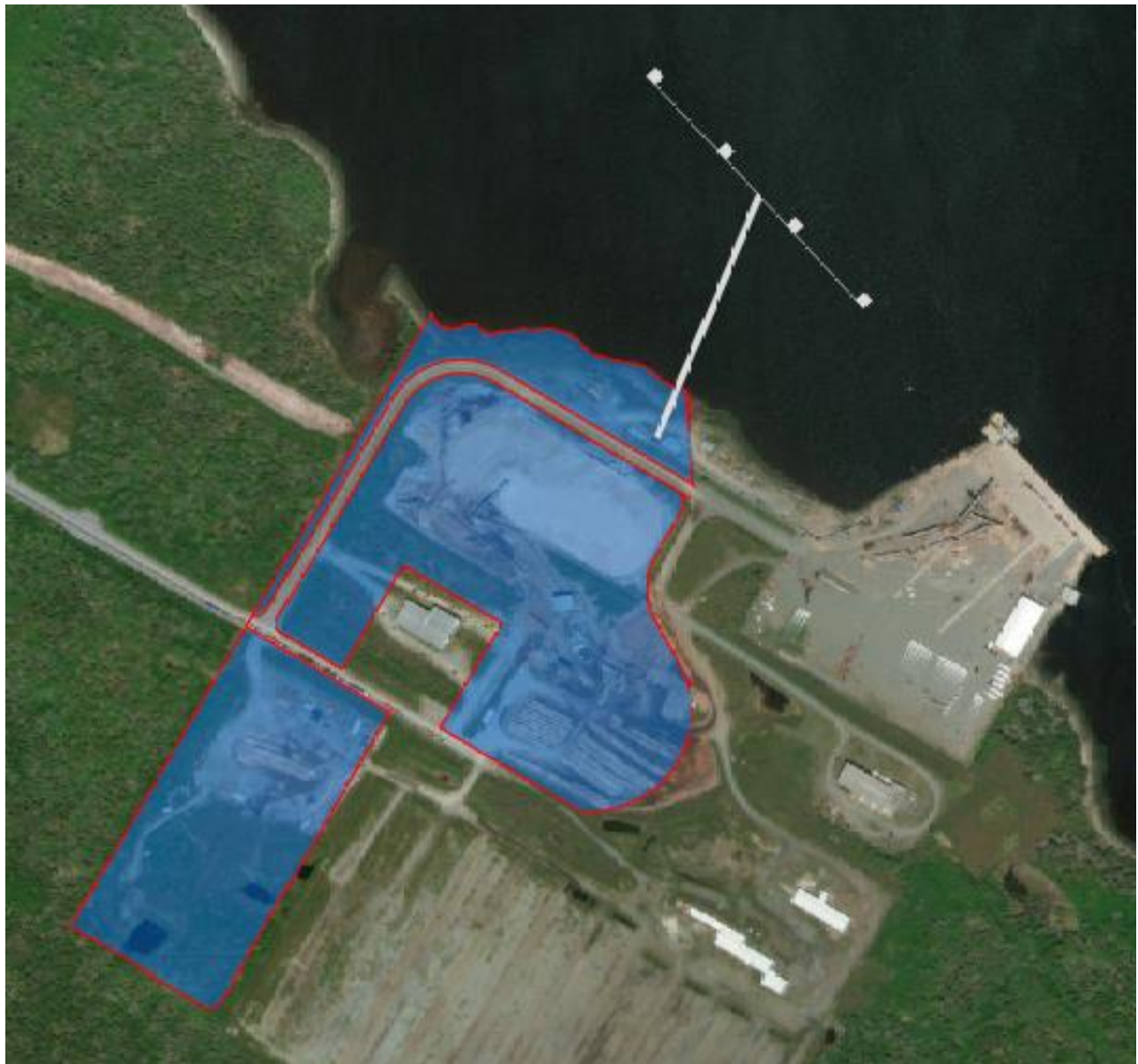
Figure 10 - West Bulk Material Handling
