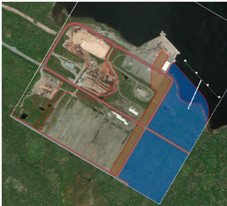
Figure 12 - East Bulk Material Handling
